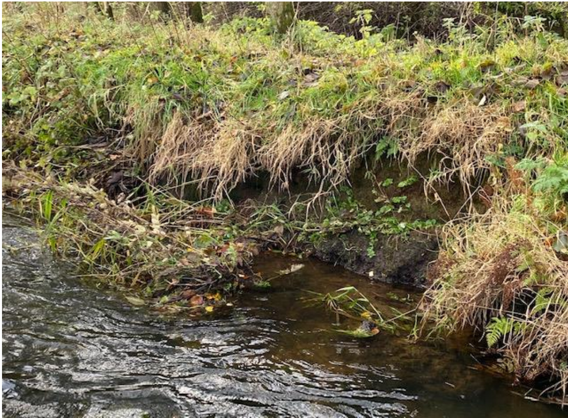
Figure 4, Ebrie burn, collapsed section below.
