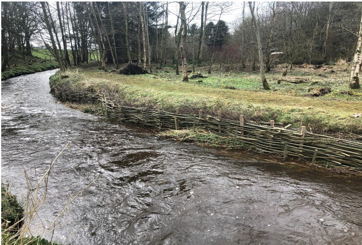
Figure 1, Willow bank repair on the Ebrie, March 2022.
